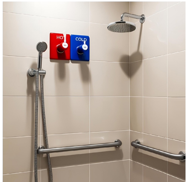
Example of a shower setup to support independent showering, including colour-coded taps, a shower hose, and handrails.
